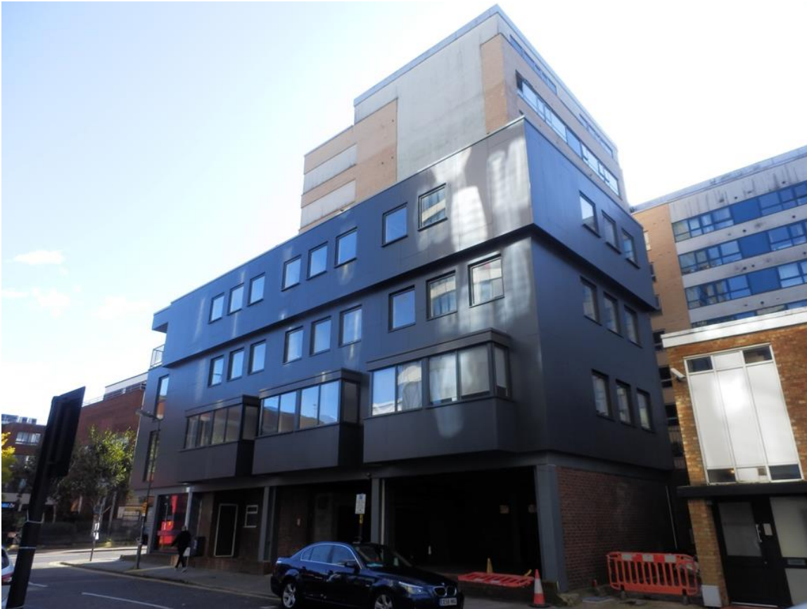
Frontage onto Junction Rd
