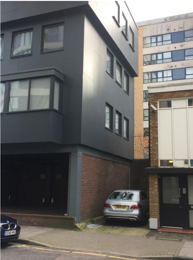
Car parked in proposed bin and cycle storage area
