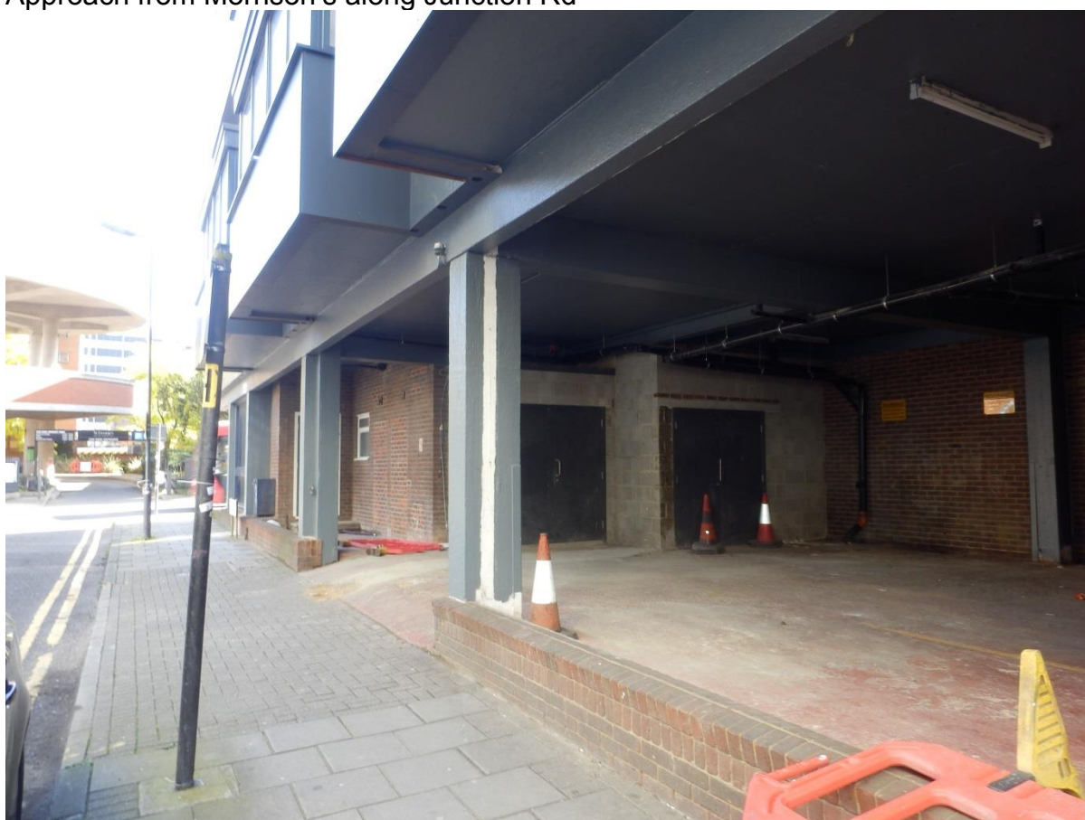
Undercroft area along Junction Rd
